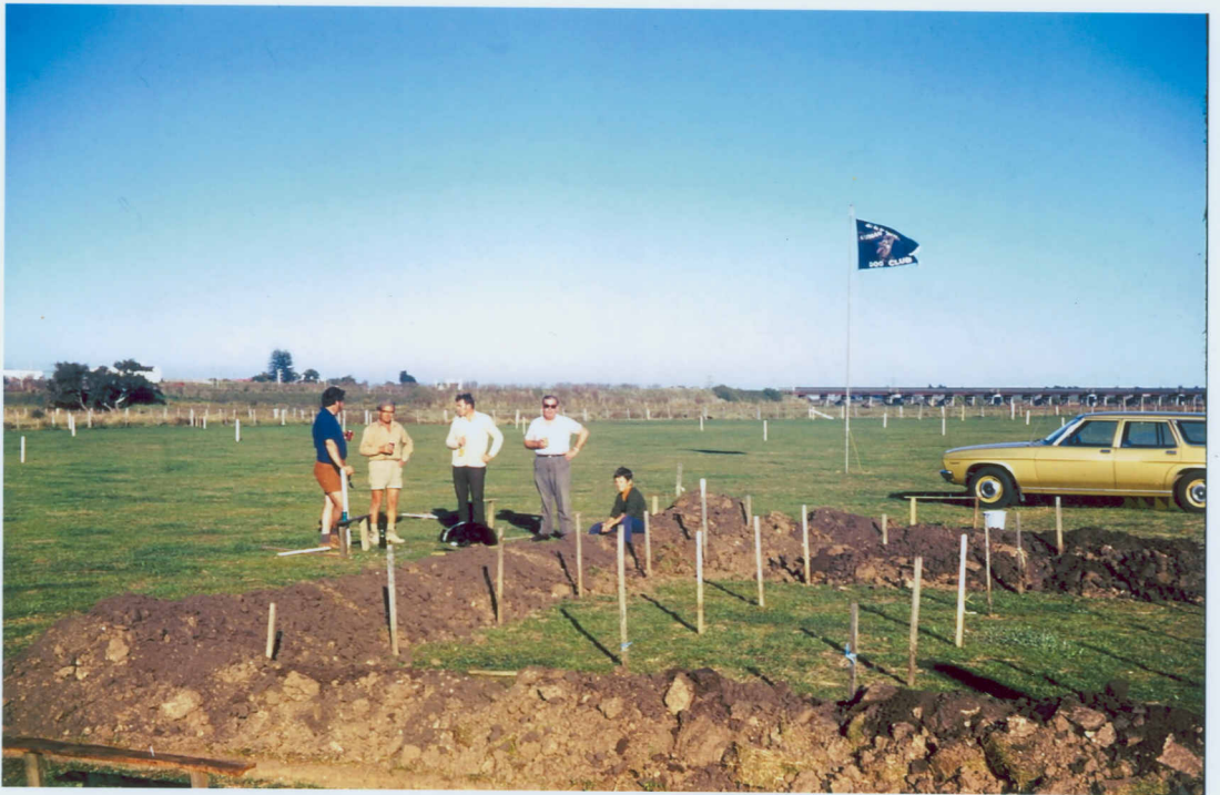
WALL FOUNDATION TRENCHES ARE DONE, STUMPHOLES TO GO
